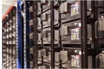
Photos: Building-integrated battery storage in Chemnitz (Left/Right: Outdoor view; Center: indoor view showing Samsung Li-Ion battery units)
